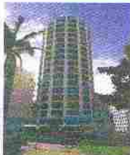
Iconic rebuild... the former Gazebo Hotel, now known as 2 Elizabeth Bay Road, with The Court next door.
